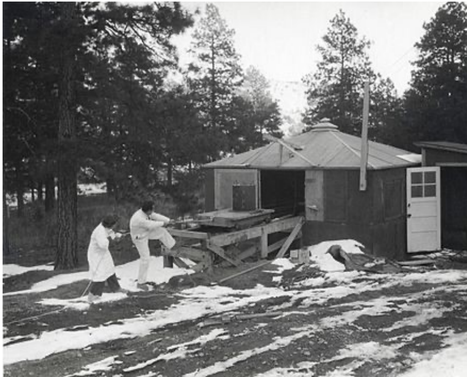
Remote handling of a kilocurie source of radiolanthanum for a RaLa Experiment at Los Alamos
