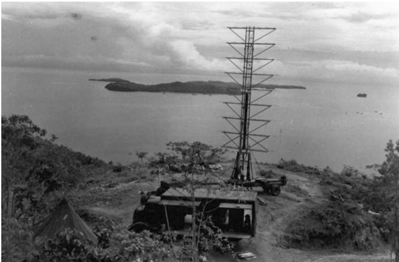
Opana Point radar station.
